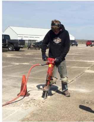
Mike Mounlio did a ton of jackhammering.
