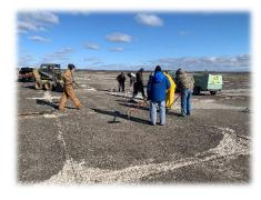
Day 2, Dig Day, was cold and windy when we brought out the heavy artillery. Jackhammers and the air compressor circulated the site and pulverized the cut areas. The
